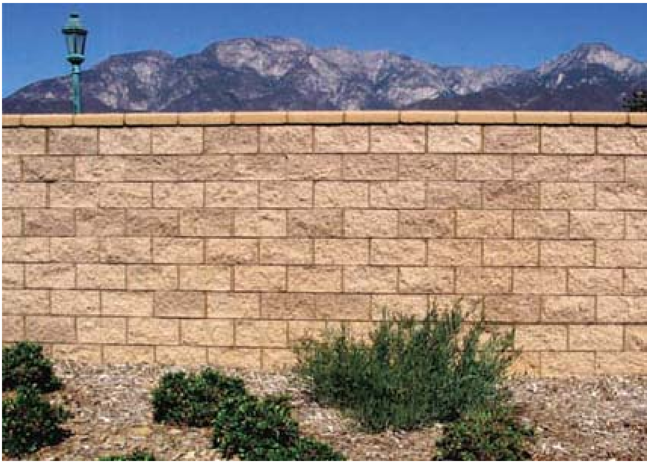
SPLIT FACE BLOCK WALL
